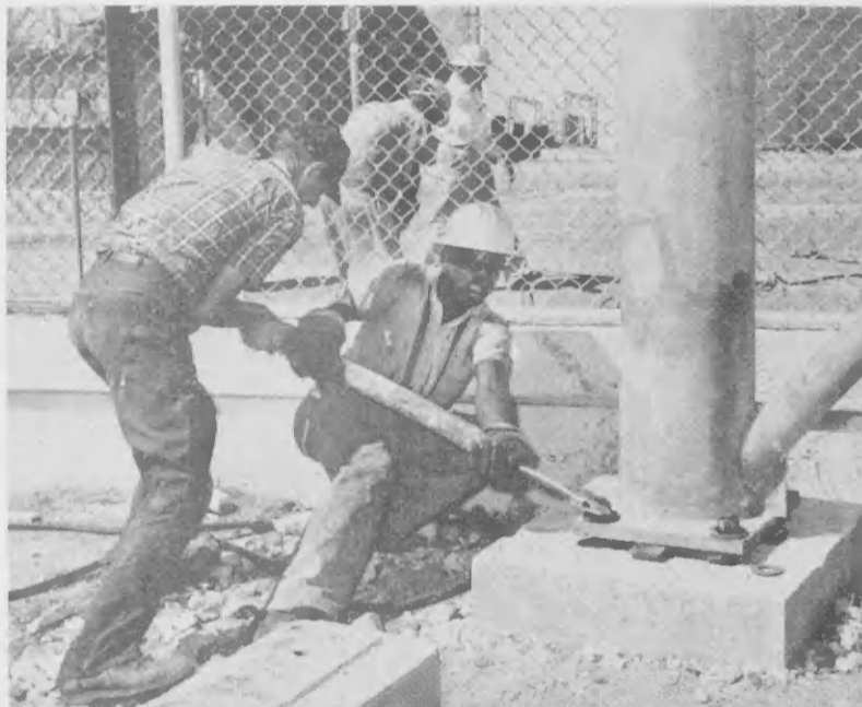
COLUMNS WERE bolted to concrete pads anchored deep in the coral, and were fabricated out of twelve-inch pipe. Workmen apply leverage to a wrench in the operation. COLUMNANAN A worde firmá cu bolt ariba plachi di concreto hanerá hundo den e coral y a worde fabricá di tubo di diez-dos duim.
